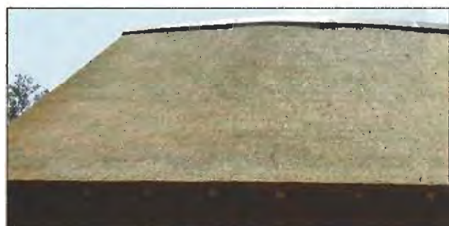
Roof slope 45 degrees
