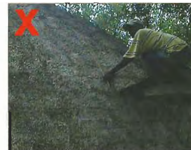
Roof's life drastically reduced due to combing without first pulling back the thatch beforehand as required
