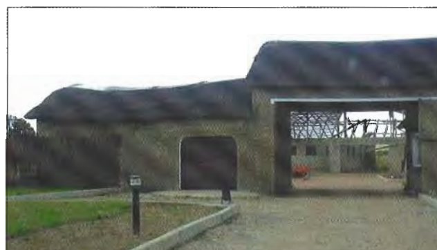
Wrong pitch and thatch layer poor
