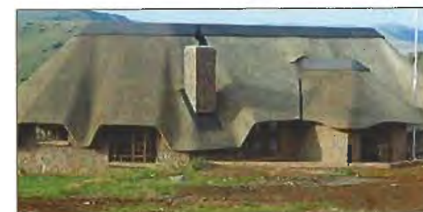
Correct chimney design
