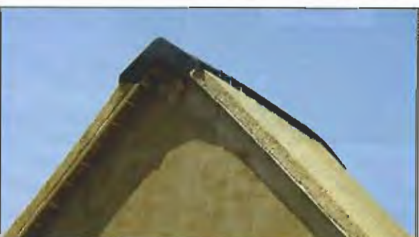
Correct installation of ridge
