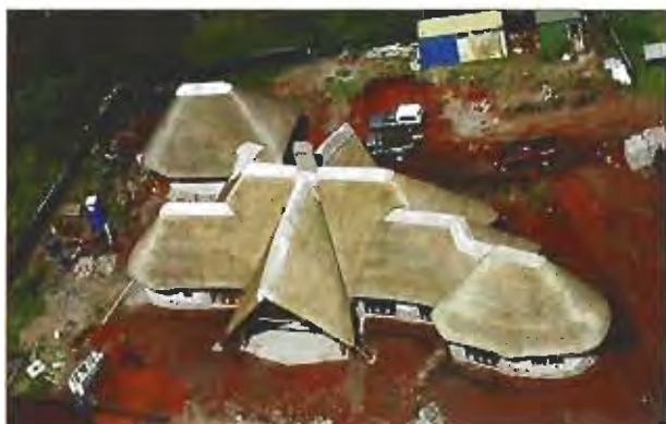
Good design. Open valleys and no overlapping of thatch surfaces
