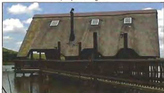
Roof slope 50 degrees
