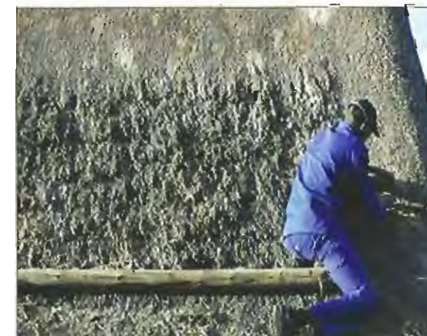
Pulling down of thatch layers.
