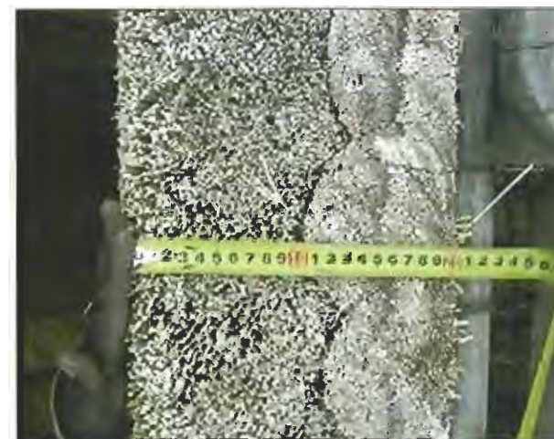
Functional thickness of thatch above sways not less than 70mm. Total thickness not less than 175mm
