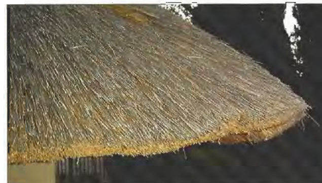
Poor compaction, loose and thin over hip
