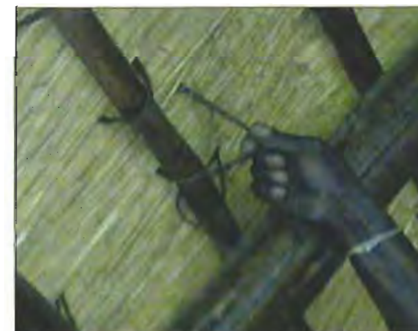
Tightening of twine after pulling down of outer layer of bundles.
