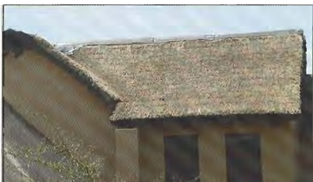
Wrong pitch and thatch layer poor
