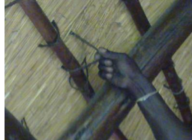
b) Twine tightening on a thatched roof
