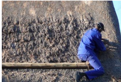
a) Pulling down of the thatch layers of a thatched roof
