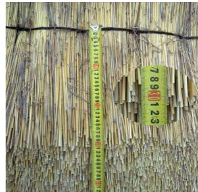
b) Thickness of the thatch for a longer life span
