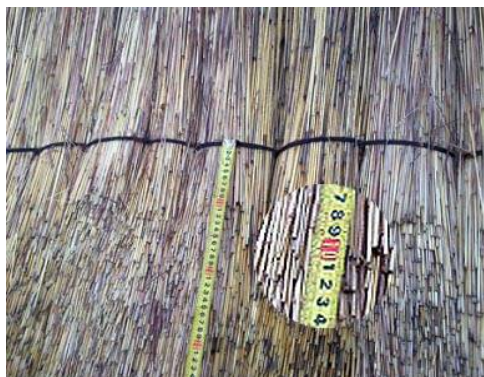
a) Thickness of the thatch for a shortened life span
