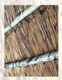
According to the SANS 10407 (Thatched Roof Construction) Specification, the only approved binding materials are stainless steel wire and tar-treated sisal twine.
