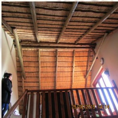
The clear span of ridge beams in the apex of the roof is 4 m where it should not exceed 3 m.
