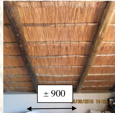
The rafter spacing is between 900 and 950 mm whereas the maximum should not be more than 800 mm.
