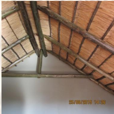
Roof built at 35 degrees
