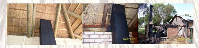
These installations above are incorrect and do not comply with regulations. The pole and thatch shows charring next to the steelflue.
