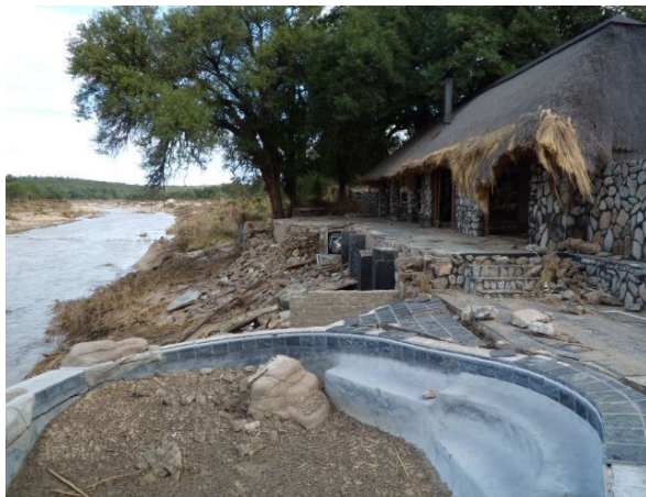
After the flood
