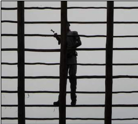
Incorrect, without safety harnesses
