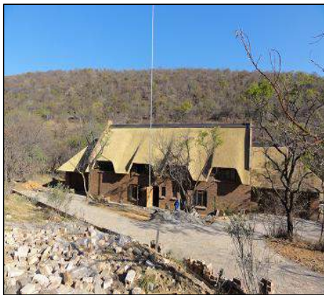
Correct installation of dormer windows.
