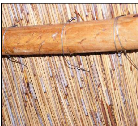
Loose wire is not tight around lath
