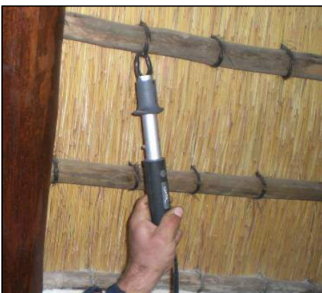
Correct binding tension.
