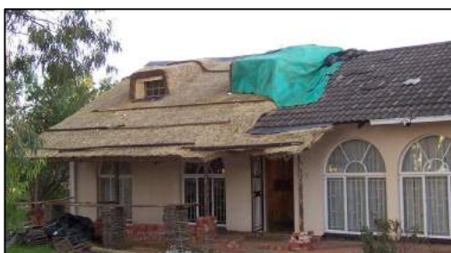
Incorrect pitch for a thatch roof.
