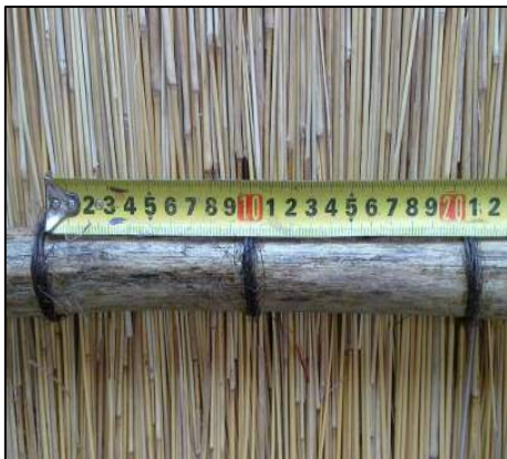
Correct binding spacing at 110mm. Note the twine is tightly around the lath
