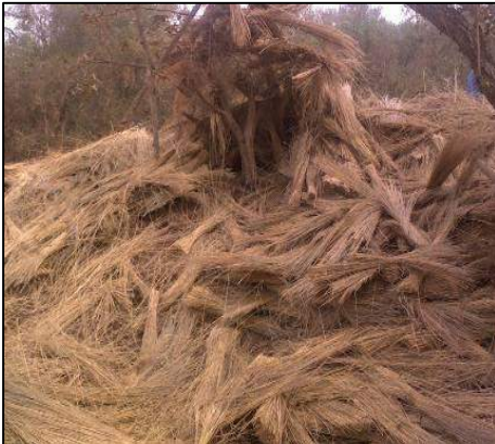
Incorrect storage of thatch grass on site
