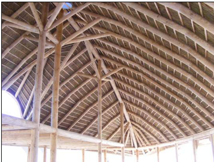
Note the Curved Rafters
