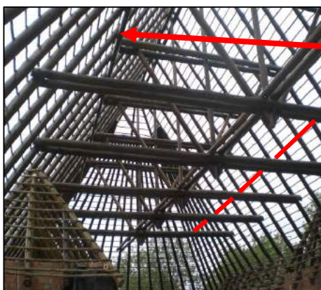
Intermediate Ringbeam Trusses spaced correctly no more than 2.700m apart.
