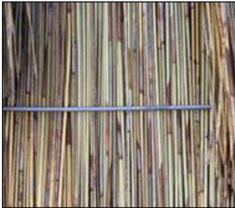
Galvanised wire sway of min 3.15mm
