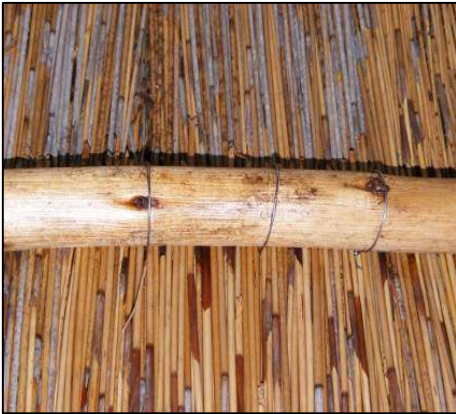
Correct wire binding tension around lath
