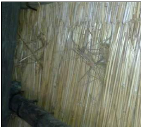
Poorly finished, seed ends are visible.
