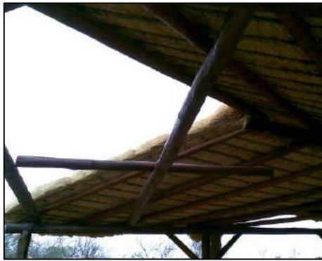
Collapsed roof structure due to no wind brace supports.
