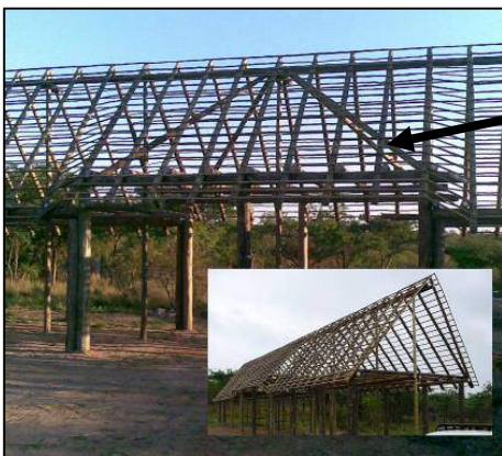
Shows wind brace support beams bolted to the underside of rafter poles.
