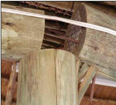
Improper ring beam connection to upright. Note only nails!
