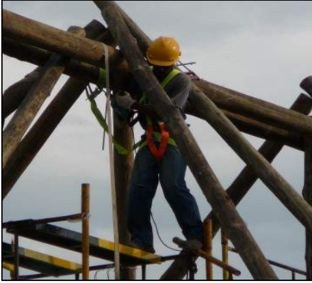
Correct, with safety harnesses
