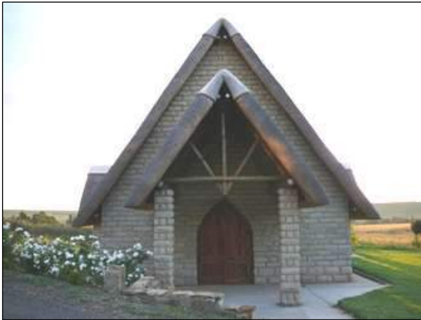
An example of rolled thatch gable ends.
