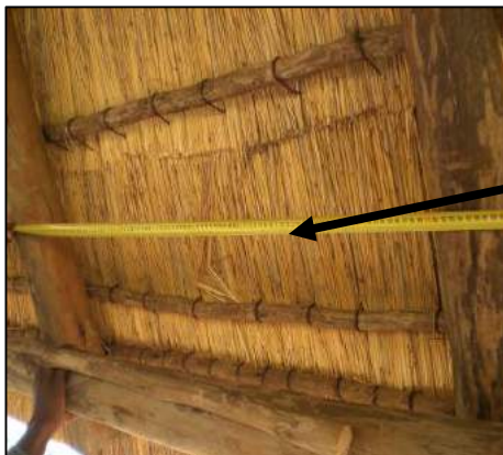
1 000 mm Incorrect rafter spacing, shows more than the allowable 900 mm centres.
