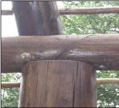
Shows example of bolting and connection of Ring Beam onto upright.
