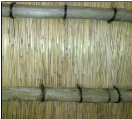
Good example butt and seed ends are not visible. The butt ends are concealed. Twine is tight around the lath.
