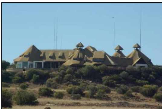
Multiple lightning conductors.
