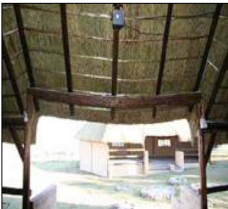
Ring beam with deflection.
