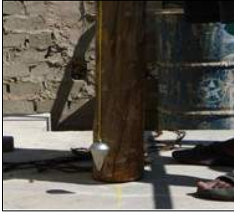
Incorrect plum bob position.
