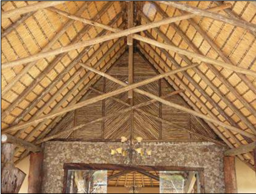
Lathe Cladding to gable walls.
