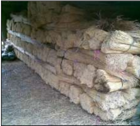
Correct storage of thatch grass on site
