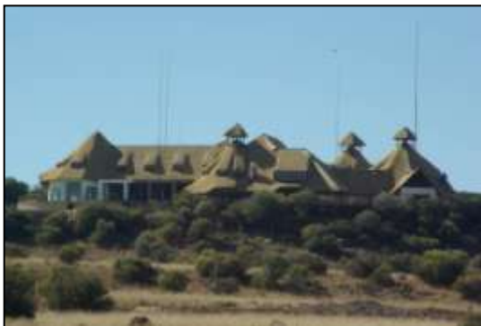
Multiple lightning conductors.
