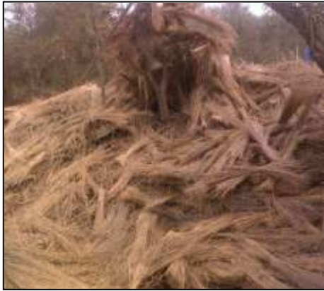
Incorrect storage of thatch grass on site
