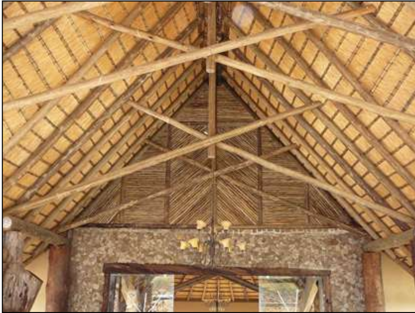
Lathe Cladding to gable walls.
