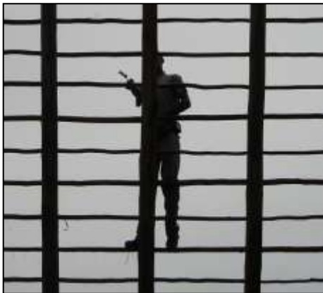
Incorrect, without safety harnesses
