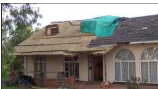
Incorrect pitch for a thatch roof.
