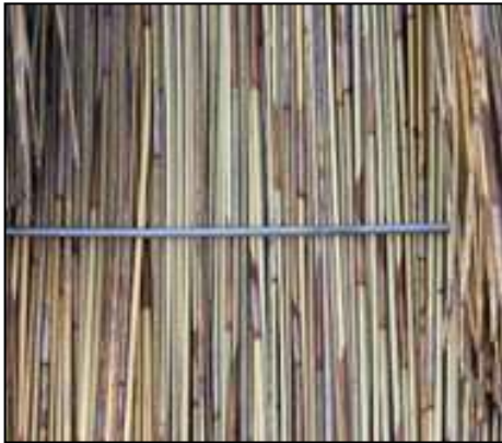
Galvanised wire sway of min 3.15mm
