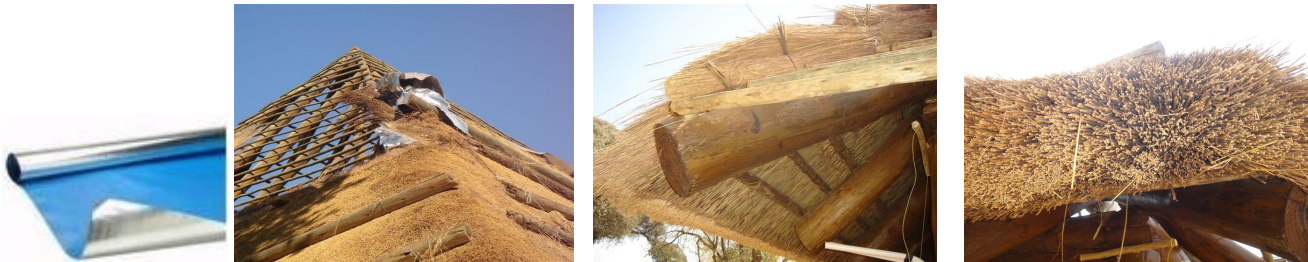
The thatch thickness is tapered down dramatically to the ridge
