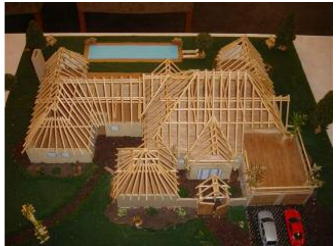
Most aesthetic pole structure. (Slope 50 degrees)
