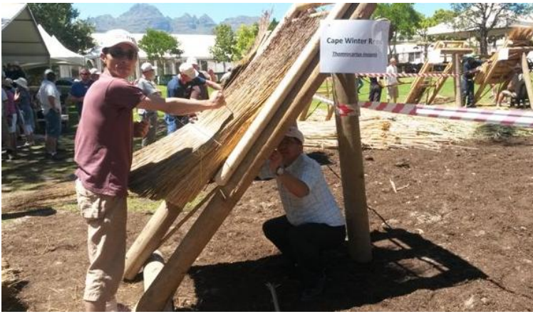
Japan demonstrated how to thatch a Japanese style roof with Cape reed
