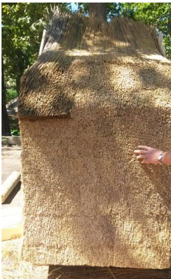
Demonstration of how to thatch a bend
