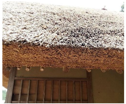
An example of the thickness of Japanese roofs
