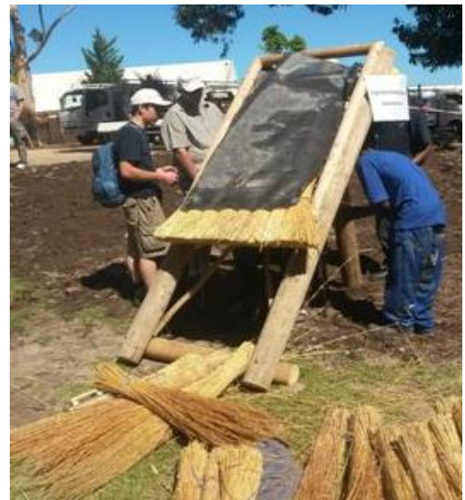
Demonstration of the installation of a fire blanket
