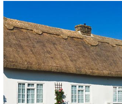
An example of the ridge detail in the UK
