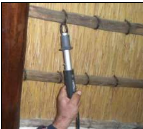
Correct binding tension.
