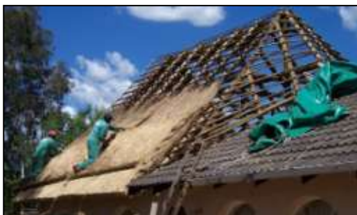
Correct pitch for a thatch roof.
