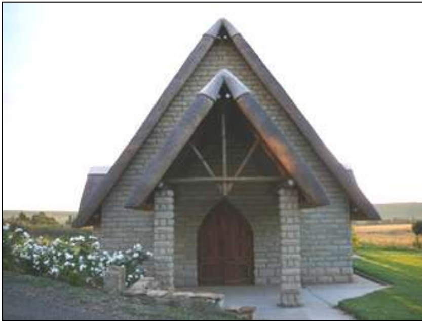
An example of rolled thatch gable ends.
