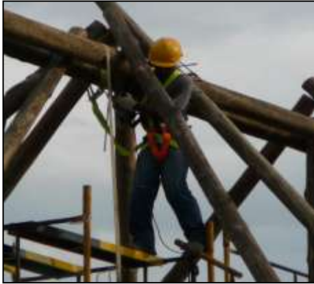
Correct, with safety harnesses
