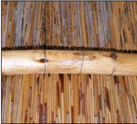
Correct wire binding tension around lath
