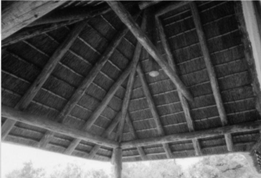
Photograph 13 Typical thatched-roof hip detail
