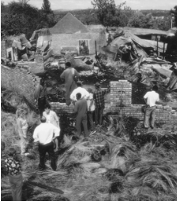
Photograph 16 Total destruction, following a thatch roof fire
