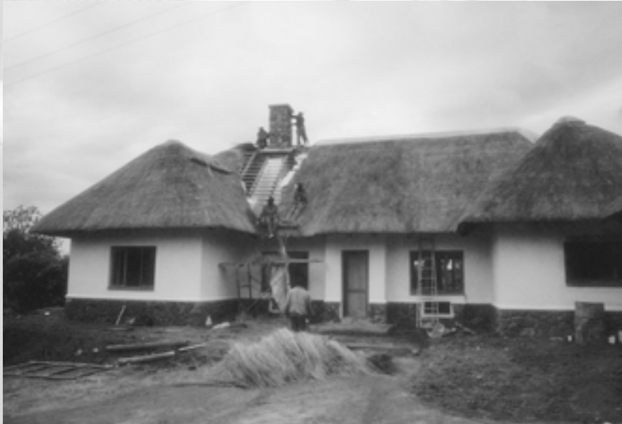
Photograph 7 Chimney (with flashings) at ridge of roof
