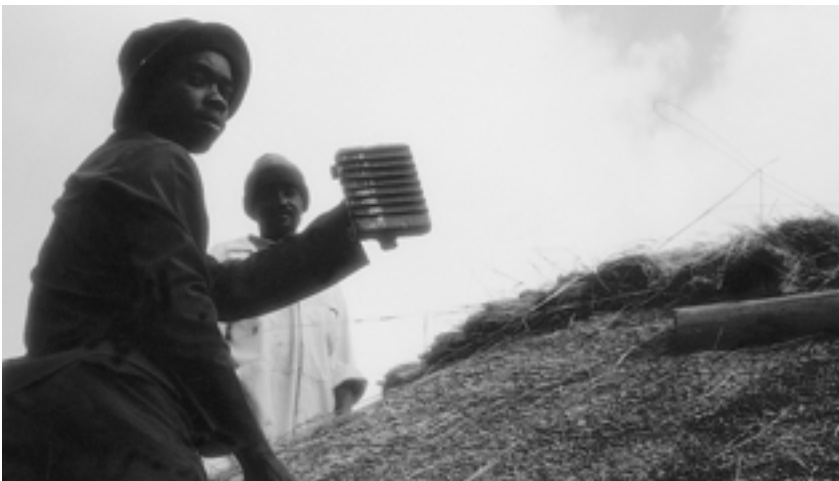
Photograph 3 Thatching spade or leggatt ("dekspaan")
