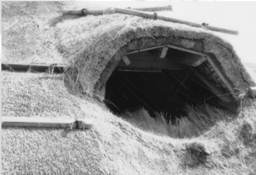
Photograph 10 Typical thatched-roof dormer window under construction
