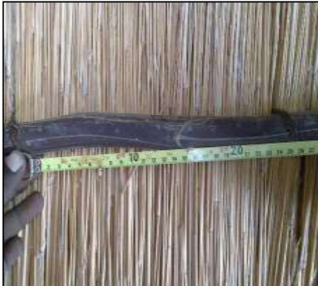
Incorrect binding spacing, greater than 110mm. Note the loosely stitched twine.
