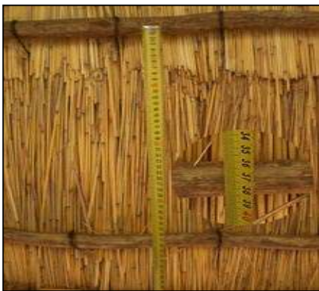
Incorrect spacing of laths as it exceeds max limit as shown in table above, also shows poor thatch finishing.
