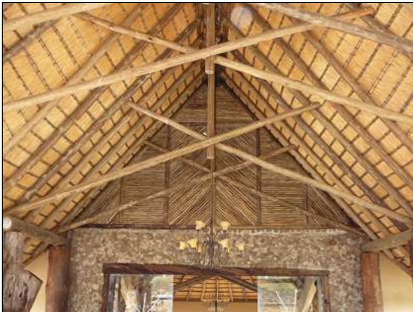
Lathe Cladding to gable walls.
