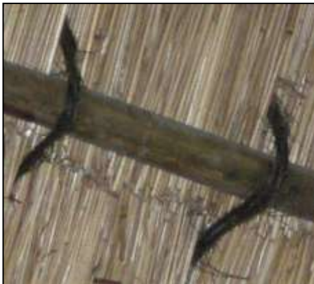
Loose twine not tight around lath which will allow the layer of thatch to slide down.
