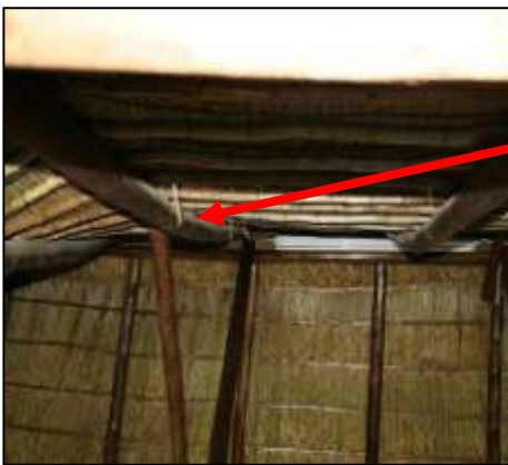
Shows deflection. Caused by thin poles and loading before tie beams are in place.
