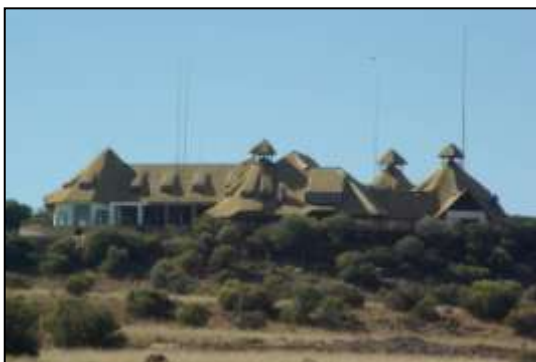
Multiple lightning conductors.
