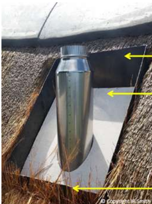
Steel shutter box
