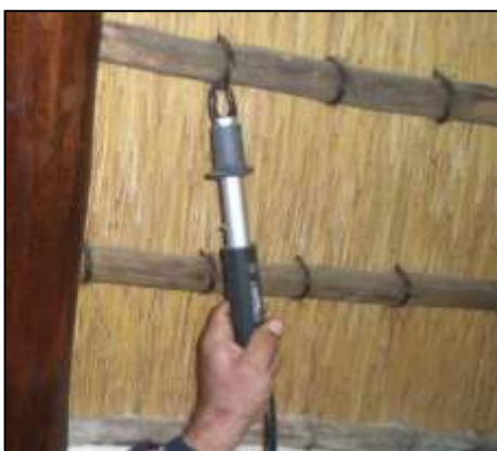
Correct binding tension.
