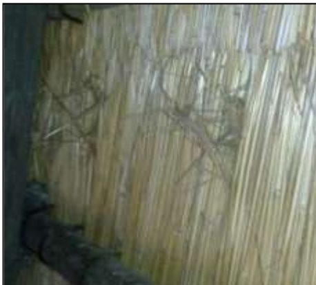
Poorly finished, seed ends are visible.
