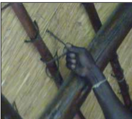
Tightening of twine after pulling down of outer layer of bundles
