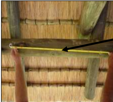
800 mm Correct rafter spacing, max is 900mm centre to centre
