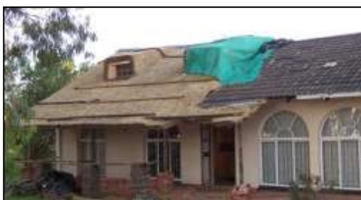
Incorrect pitch for a thatch roof.
