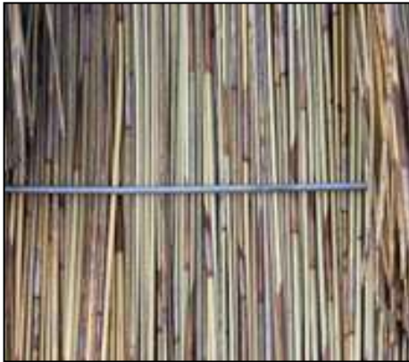
Galvanised wire sway of min 3.15mm
