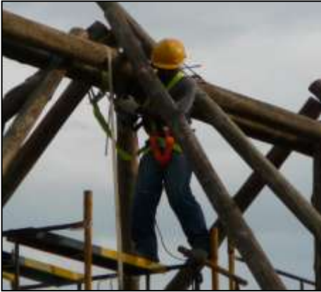
Correct, with safety harnesses
