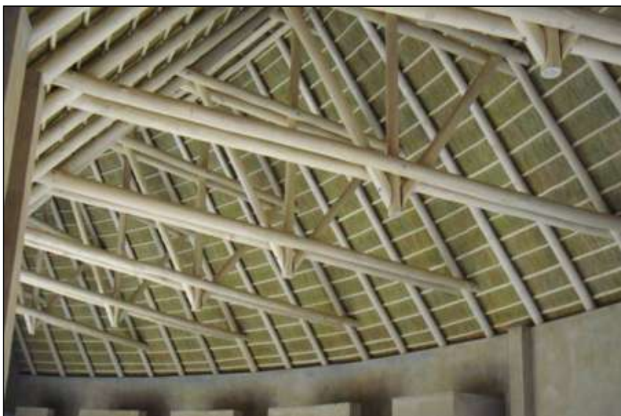
Spectacular structure on a curved building with beautiful finishing.
