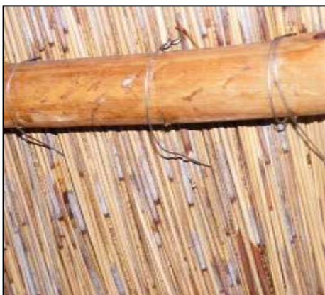
Loose wire is not tight around lath
