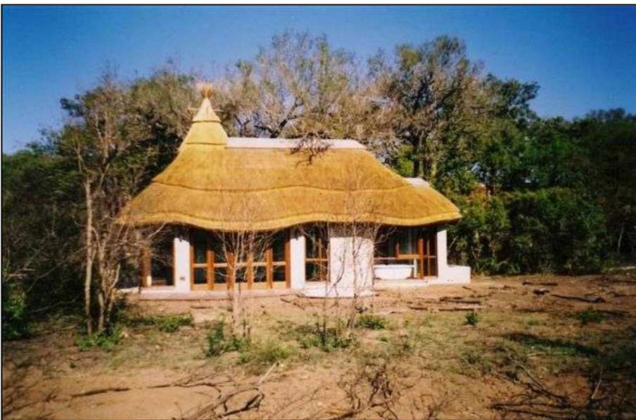
A thatch roof with rustic finishes.
