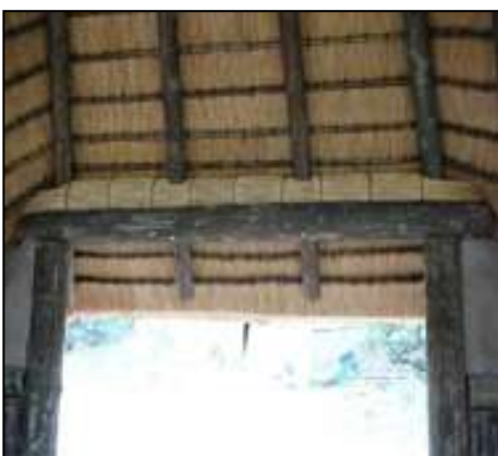
Ring beam without deflection.
