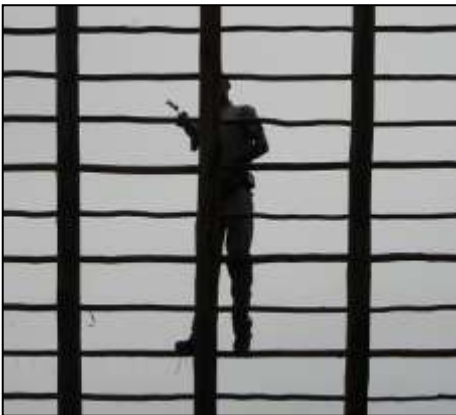
Incorrect, without safety harnesses
