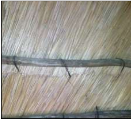
Poor finish to spreij layer butt ends not concealed by batten or laths. Note loose binding twine.
