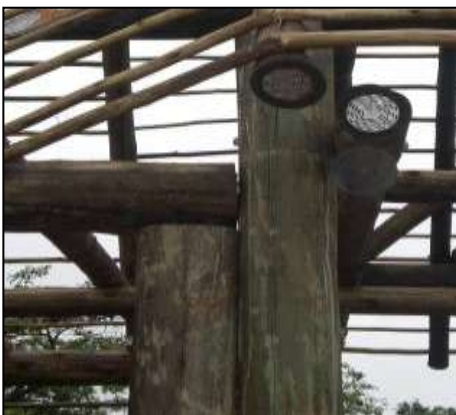
Shows an additional upright, which supports the lower ring beam.
