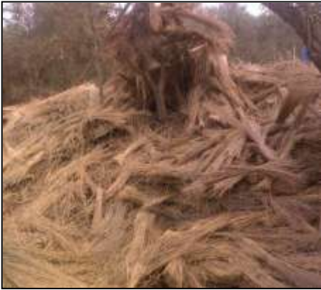
Incorrect storage of thatch grass on site
