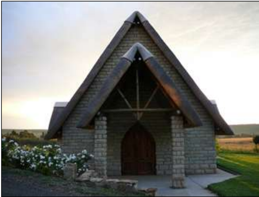
An example of rolled thatch gable ends.
