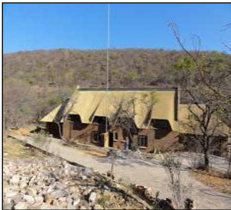
Correct installation of dormer windows.
