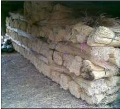
Correct storage of thatch grass on site
