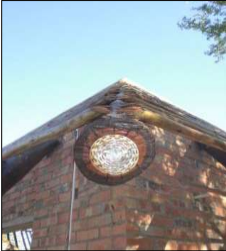
Shows no deflection on 14m pole. Long spans during construction need to be supported to alleviate deflection.
