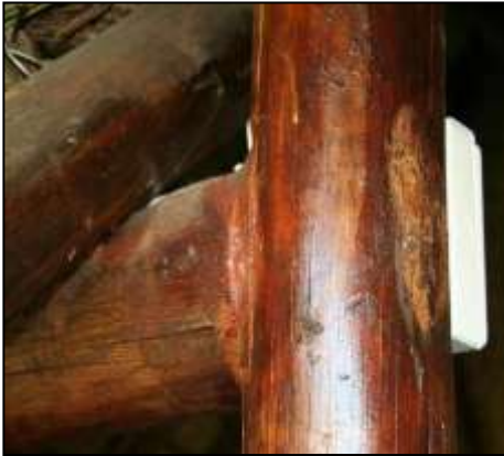
Shows poor connection of ring beam to upright.
