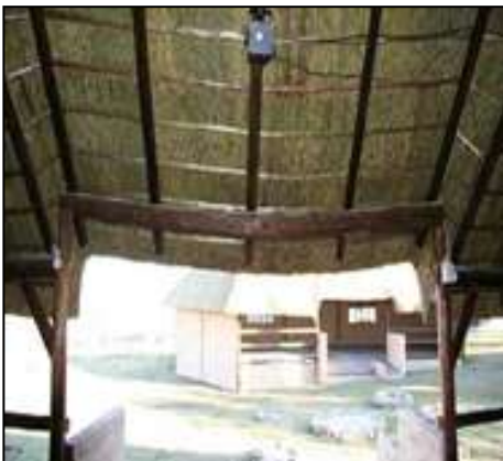
Ring beam with deflection.
